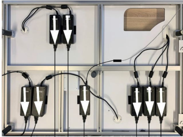
Figure 2–14: Arranging the cables
