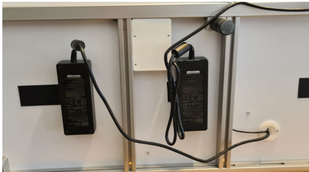
Figure 2–12: Installing the Andrew+ power supply
